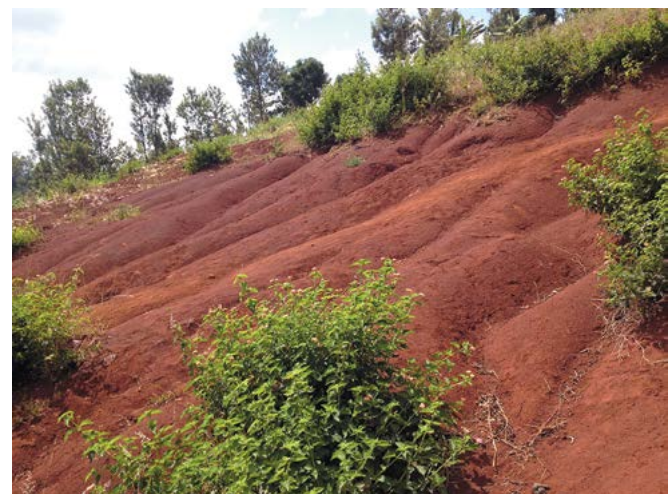
Figure 5 Erosion on a steep slope in the Upper Tana
